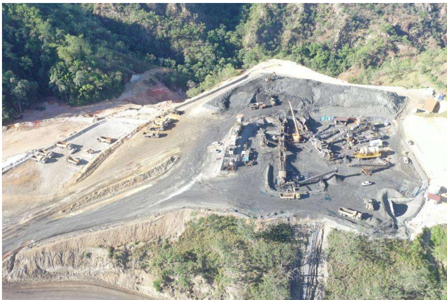
Figure 2: Aerial view of ore crushing area at Wetar
