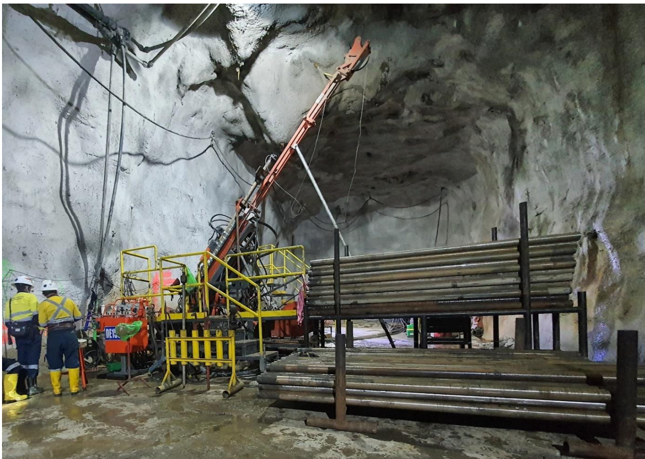
Figure 1: Underground drilling operations at Tujuh Bukit Copper Project
