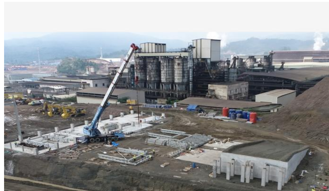
Construction of MTI concrete batching plant
