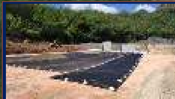
HDPE lining underway
