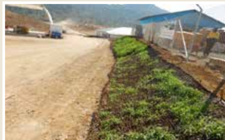
Tanaman penutup di sekitar area konstruksi Cover crops around construction area
