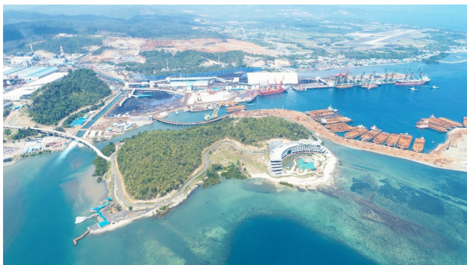
Figure 4: Aerial view of IMIP
