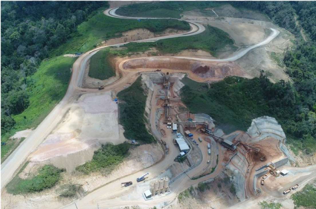
Figure 2 - Aerial view of the Ore Preparation Plant
