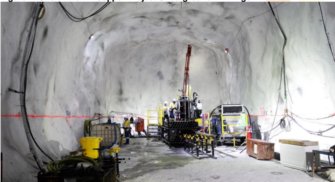
Figure 1: One of the TB Copper Project Underground Drill Rigs
