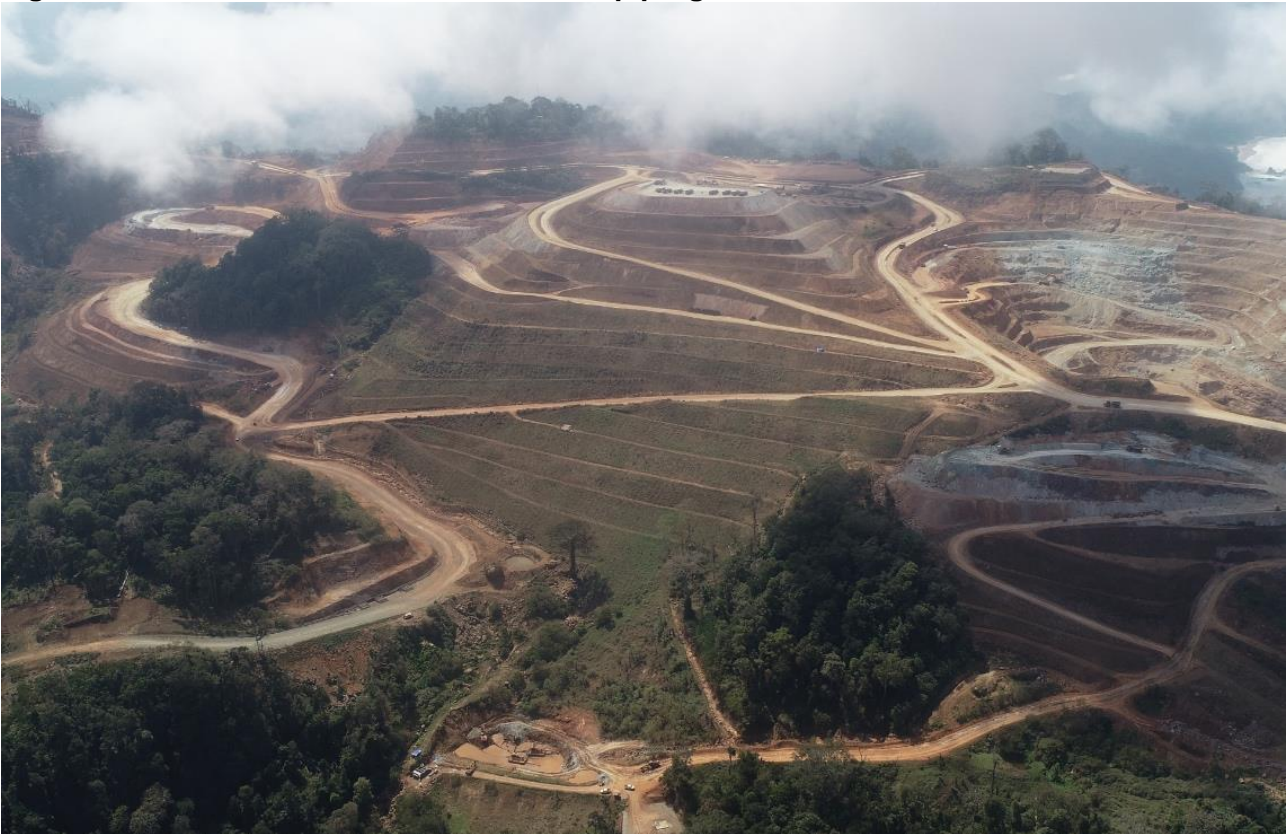
Figure 6 – Aerial view of the Heap Leach Pad showing Lift 5 in progress.
