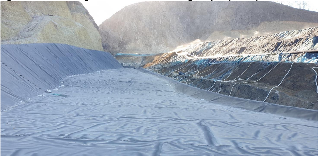
Figure 6 – Photo showing re-mining and extension to the GPLP pads for Lerokis ore.
