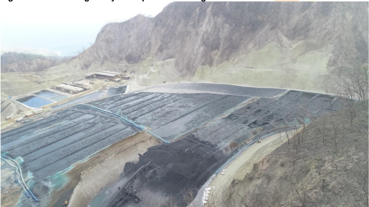
Figure 4 – Kali Kuning Valley leach pads under irrigation.
