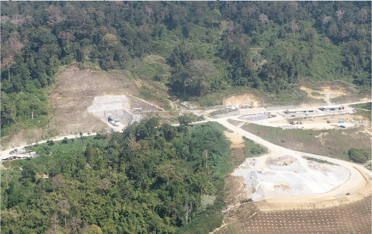
Figure 7 – Boxcut with Exploration Decline and underground infrastructure facilities.
