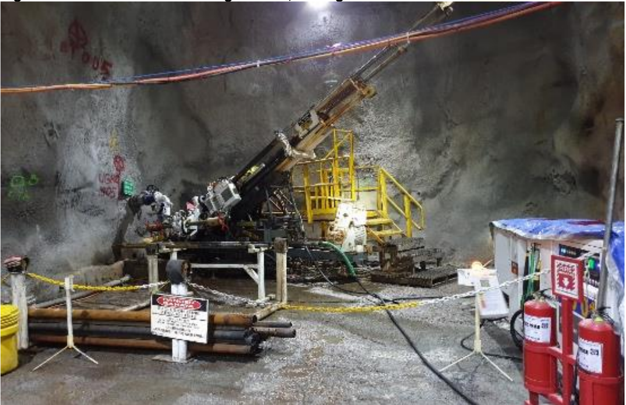
Figure 8 – LM110 diamond drill rig at SP05, drilling UHGZ-19-001.
