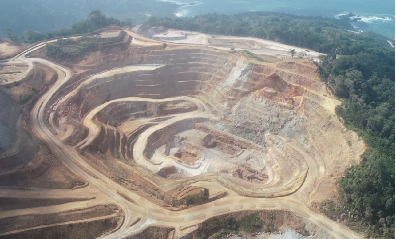
Figure 1 – Open pit mining – Pit B West showing phase 3 in the foreground and phase 4 on left side.
