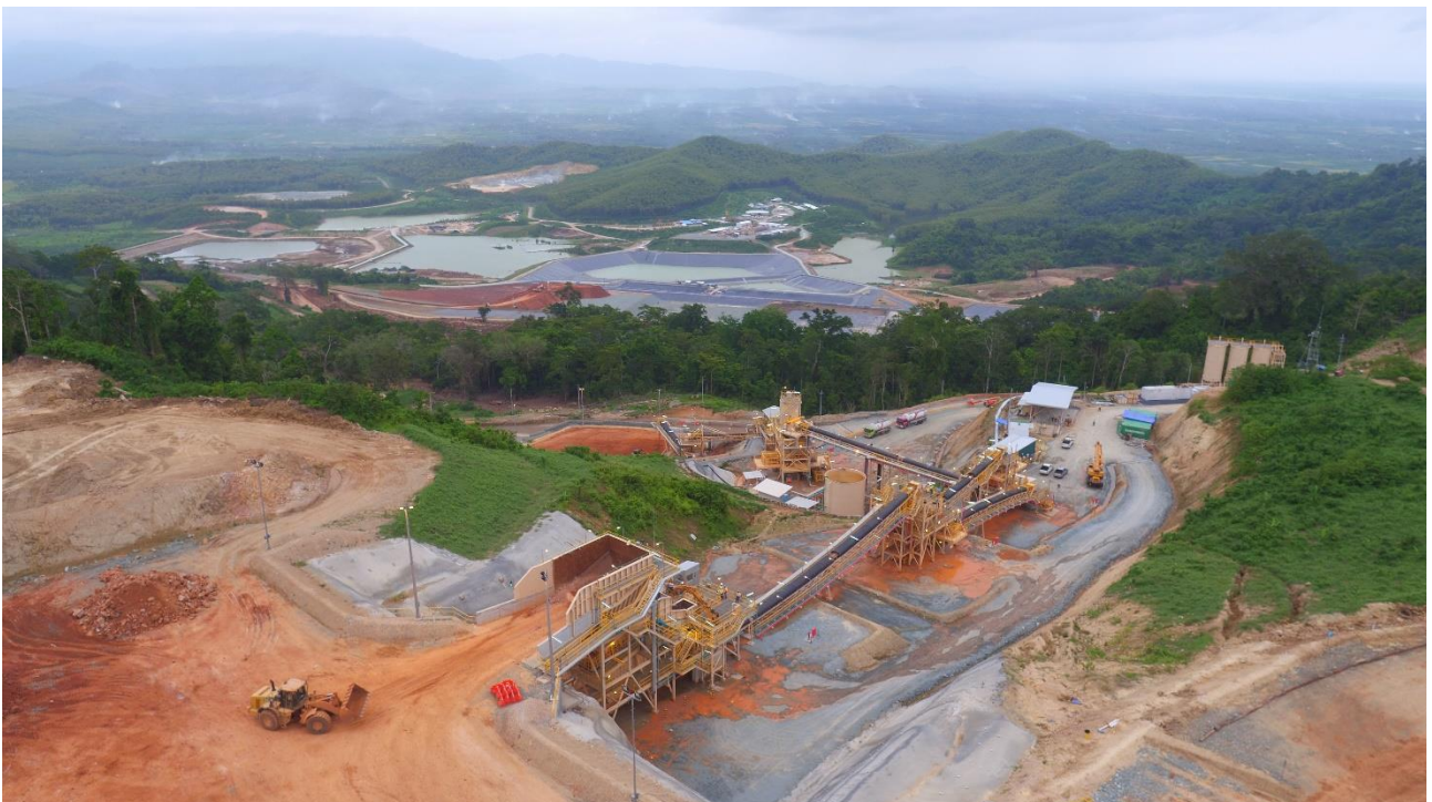
Figure 2 – Aerial view of the Ore Preparation Plant (OPP) with heap leach pad and ADR plant in distance.
