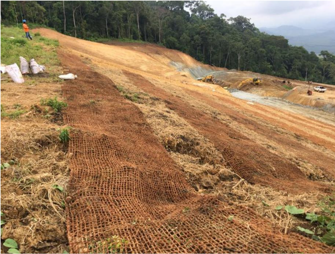
Figure 5 – Before and after pictures showing rehabilitation progress.
