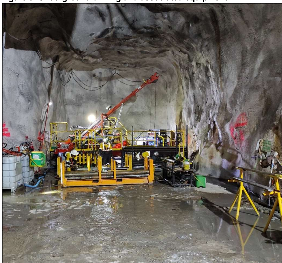
Figure 3: Underground drill rig and associated equipment
