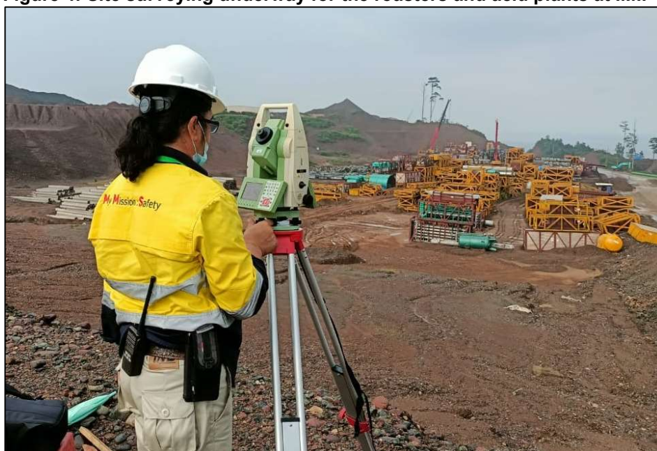
Figure 4: Site surveying underway for the roasters and acid plants at IMIP
