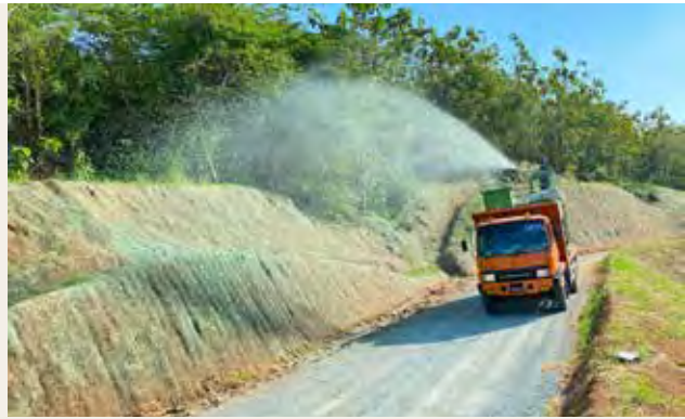
Jute Net Installation (left) and Hydroseeding (right)
