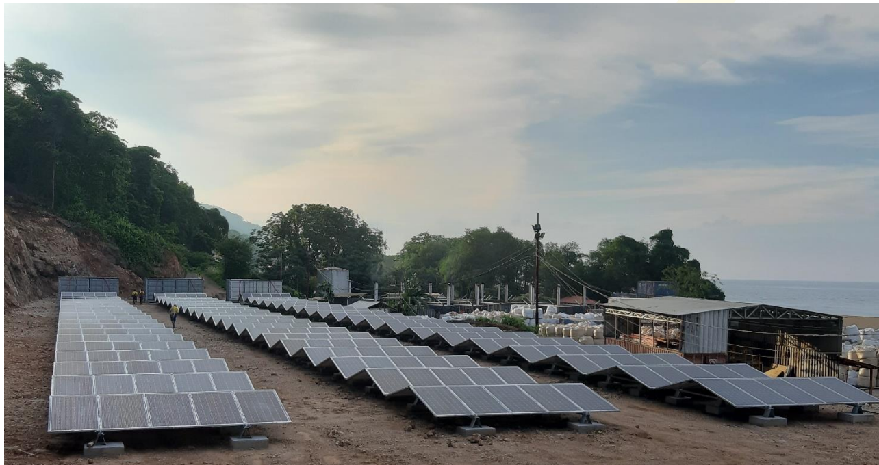
Figure 10: Installation of solar panels at Wetar
