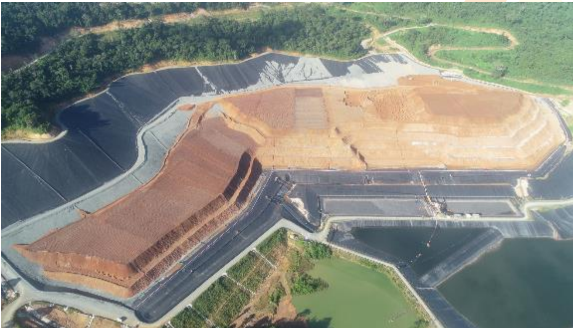
Figure 6 – Aerial view of the Heap Leach Pad showing Lift 5 in progress.
