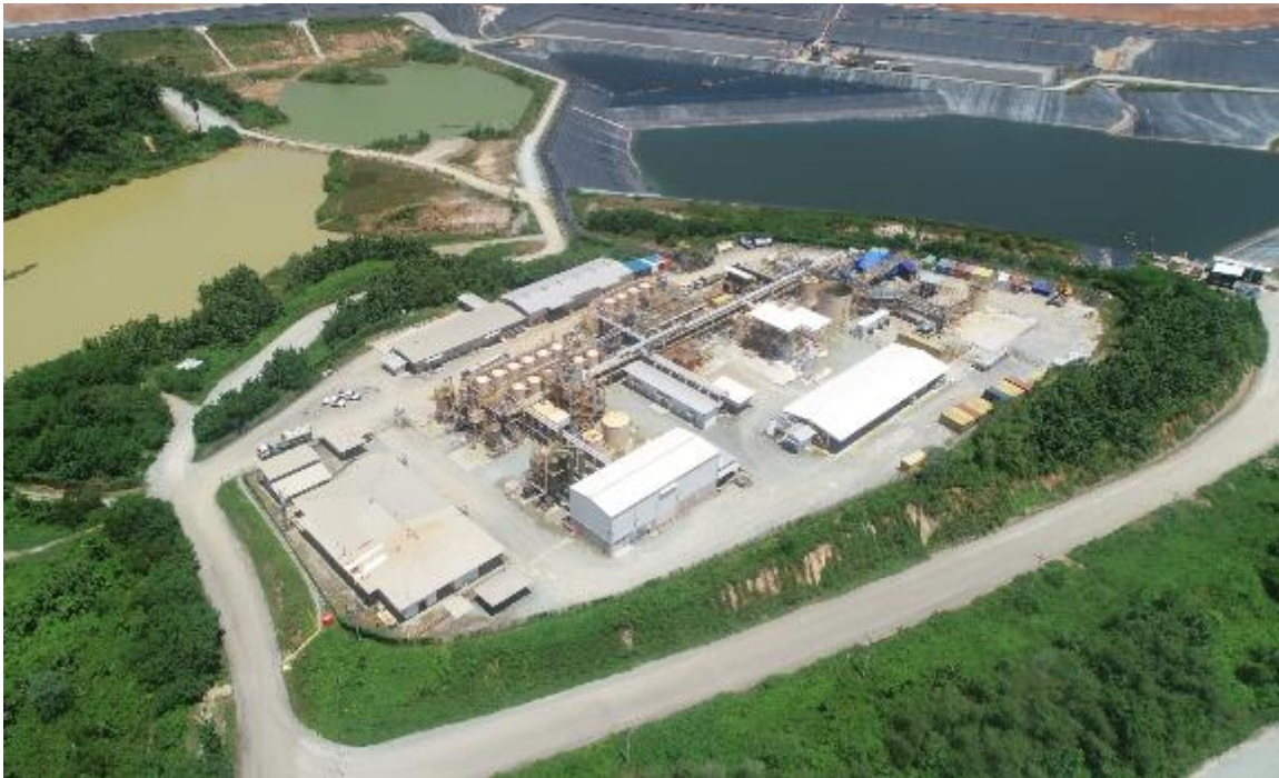
Figure 9 – ADR Plant Upgrade CIC-2 on progress.
