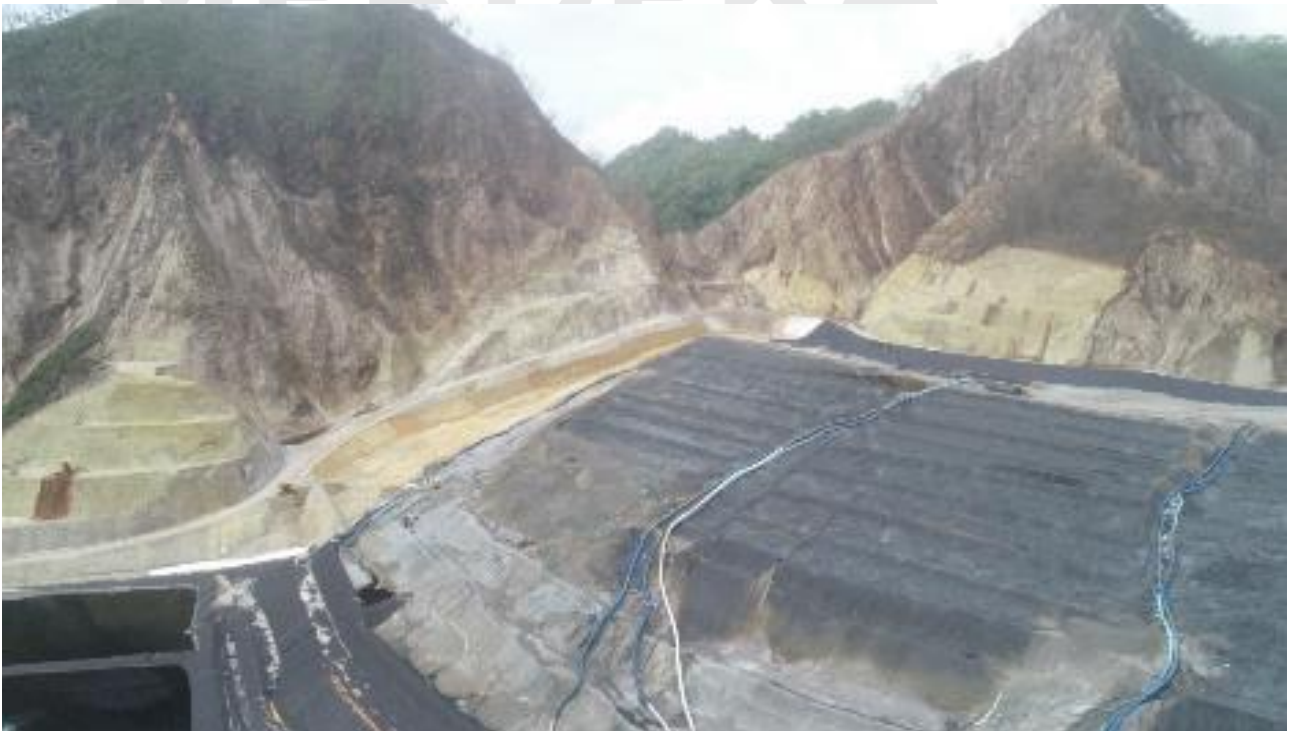
Figure 2 – Kali Kuning Valley leach pad KK01 extension progress.
