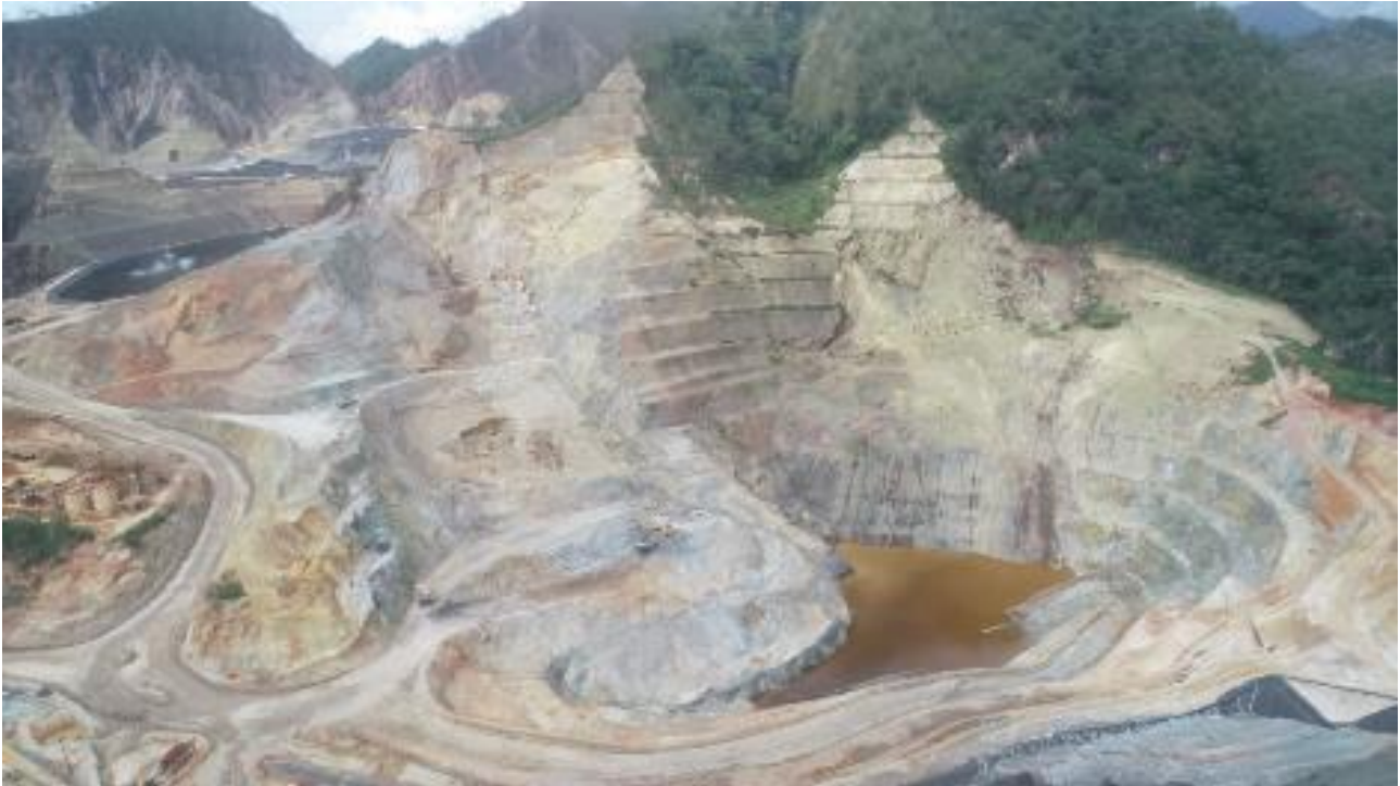
Figure 1 – Kali Kuning pit as at 31 March with pit wall remediation works advancing.
