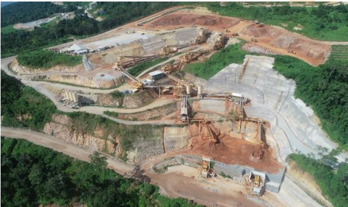
Figure 8 – Completion of OPP-2 Crushing facilities.
