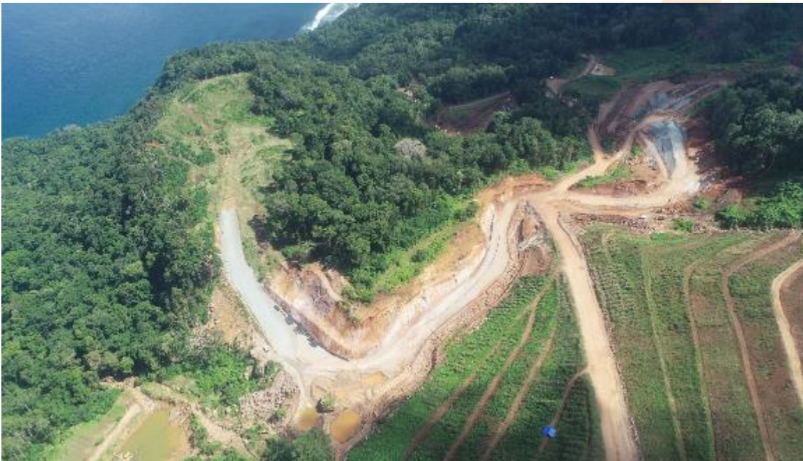
Figure 4 – Aerial view of partially cleared Pit C and haul road.
