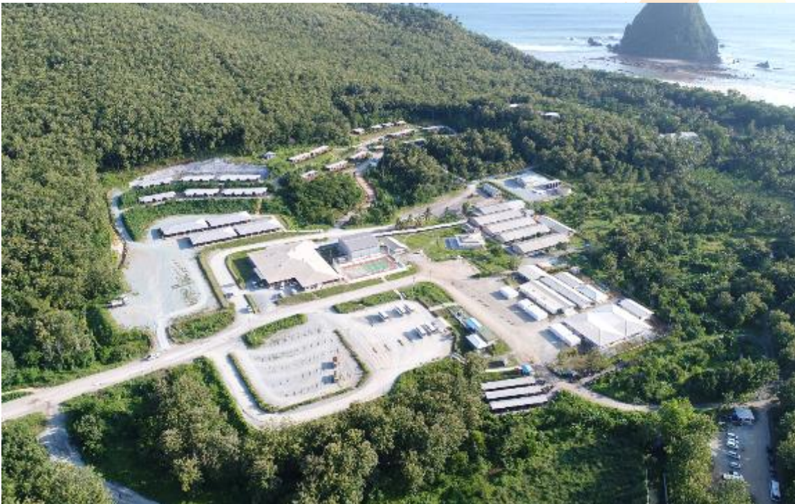
Figure 10 – Permanent Camp Expansion.
