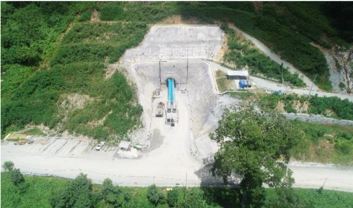
Figure 7 – Boxcut with Exploration Decline and underground infrastructure facilities.
