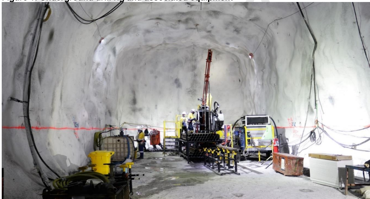
Figure 1: Underground drill rig and associated equipment
