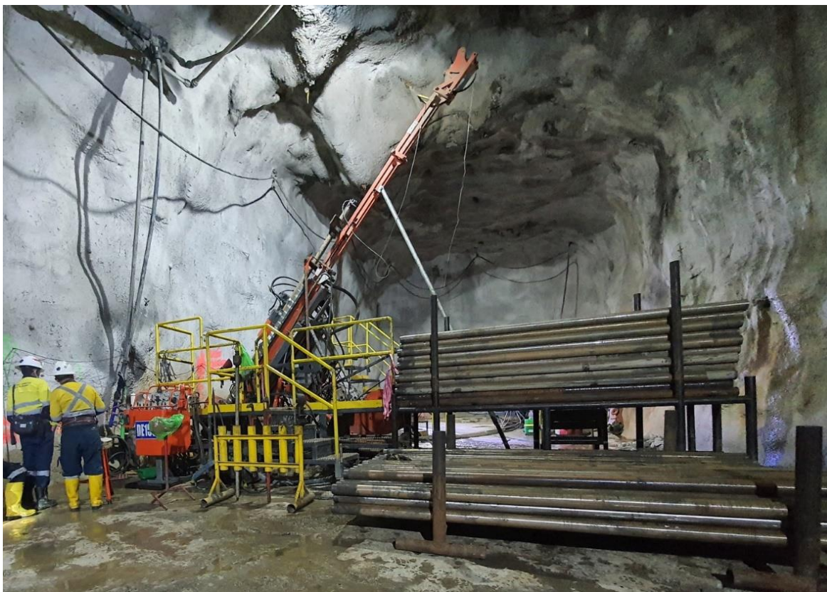
Figure 2: Underground drill rig and associated equipment
