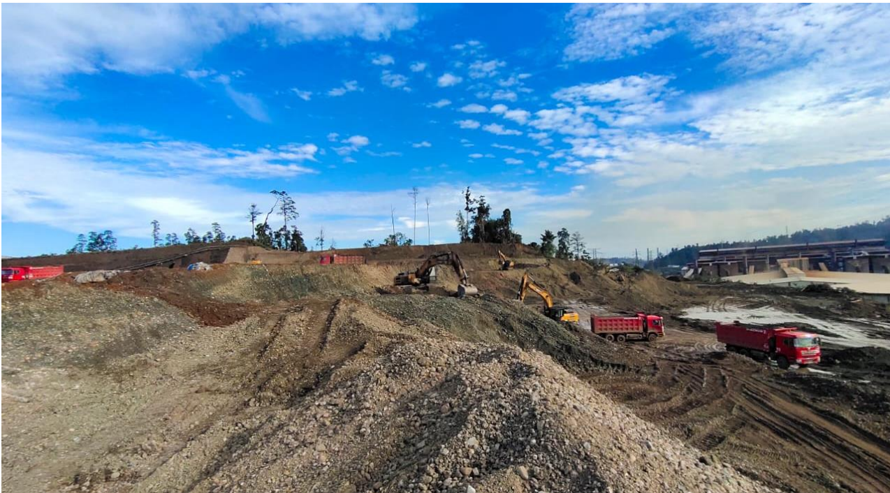
Figure 3: Ongoing earthworks in the Pyrite Concentrator Plant Area at IMIP
