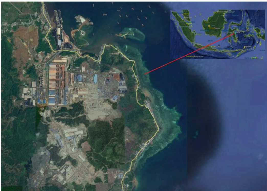
Figure 8: Aerial view of IMIP
